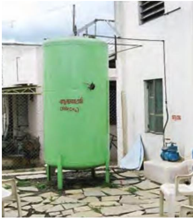
Picture 20: Gas tank in India with 10 bar pressure (photo: Sandec).
