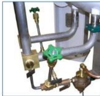
Long-life extended stem packing pressure builder and economizer isolating valves are standard on the VS-01 series.
