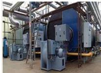
Combustion fan with frequency variator for gas / oil burners
