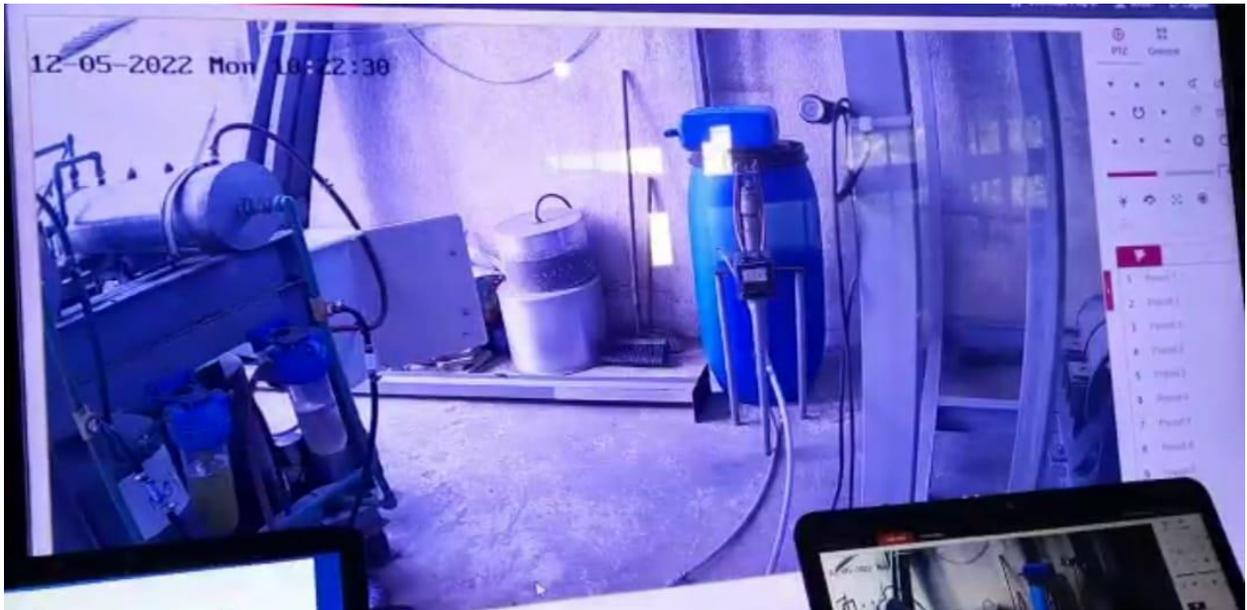
After changing the 4 tanks, we made Nitrogen purging to test the new ones. The results were also negative and the new ones didn't work well. we have leakages.
