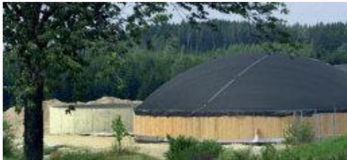
*Rubber membrane to maintain the biogas*
